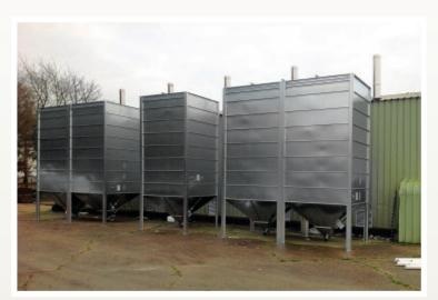
Some of the silos were installed to feed various containerised biomass boiler plant rooms which were installed on the farms, while others were feeding boilers housed inside purpose built boiler sheds, the chicken sheds themselves.
